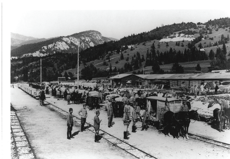
Figure 2. The first station of the narrow gauge horse-drawn railway in Bohinjska Bistrica. Courtesy of the National Museum of Contemporary History, Slovenia.
